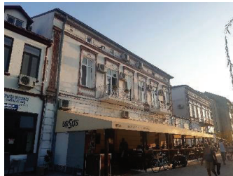
Figure 10. Sulina, Buildings on the Danube Cliff
